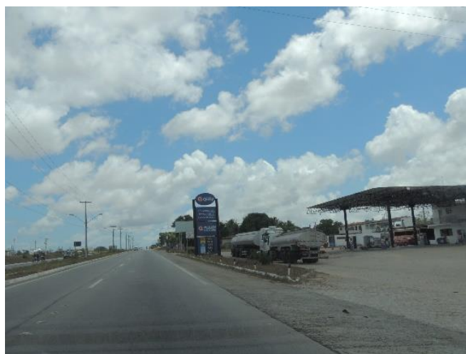
Figura 36 – Rodovia federal BR-406.
